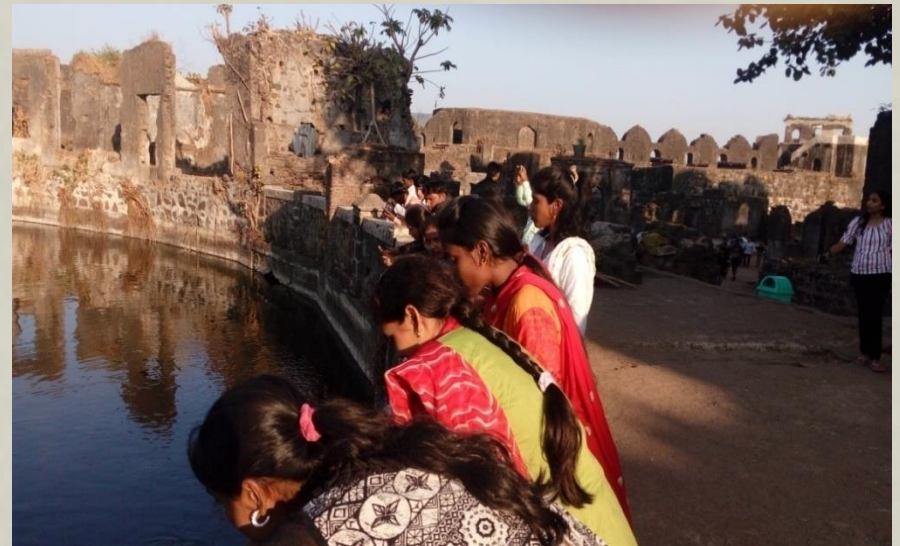
Murud Janjira Fort, water Tank
